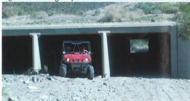
Breaking out of the tunnel
